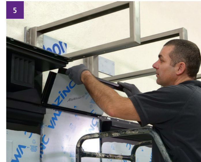
5 The inner corner panel are mounted.
