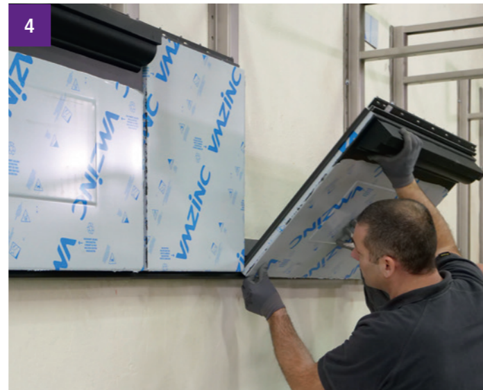
4 The cassettes are delivered with the pre-mounted decoration and are, easily self-wedging to facilitate cassette interlocking and optimize installation speed.
