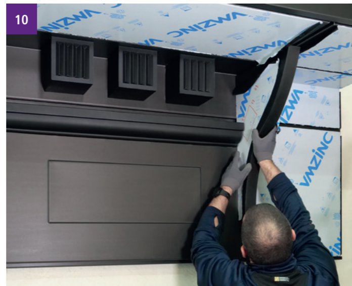
Decorated joint caps are available to hide panels and to offer vertical ornamentation.
