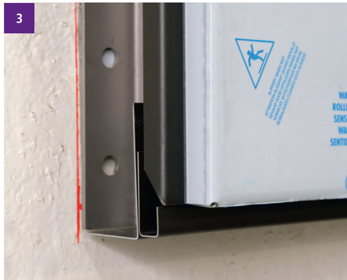
3 Install the bottom cassette into the bottom flashing, further installation from left to right and from bottom to top.
