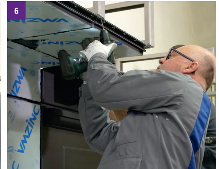
6 The cassettes are fastened to the Omega rail using the self-drilling screws.
